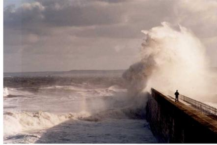
**Figure 1.1:** Violently overtopping wave at a sea wall. Picture by G. Motyker, HR Wallingford.
