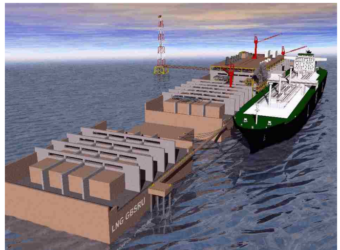
Figure 1: Gravity Based Structure as LNG import terminal
